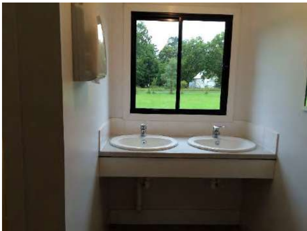
Hand basins in bathroom
